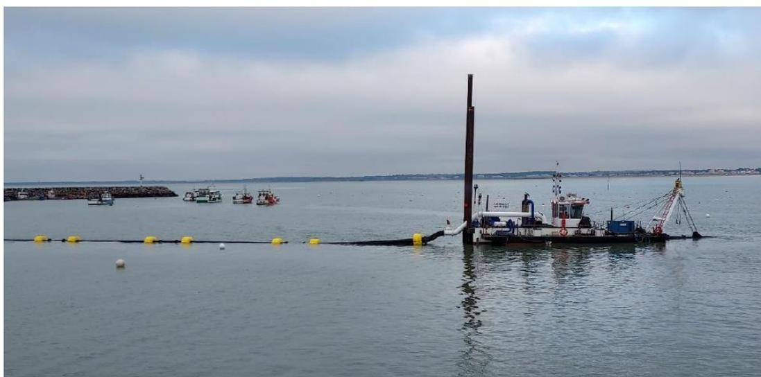
**FIGURE 11 – DRAGAGE HYDRAULIQUE PAR DAS AVEC CANALISATION FLOTTANTE (EGIS, 2022)**
